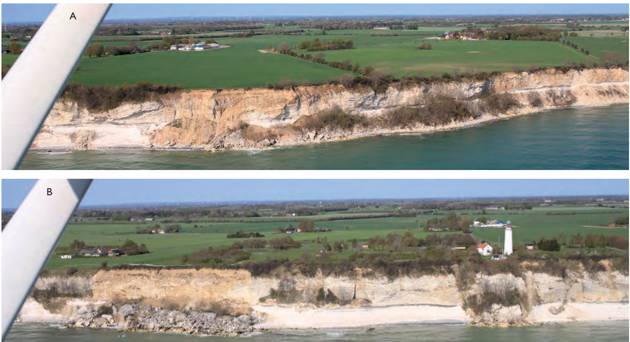
Fig. 5. Cliff sections showing various types of rockfalls at Stevns Klint. A: Cliff slide at Tømmestrup. B: Cliff fall at the lighthouse of Stevns Fyr.
